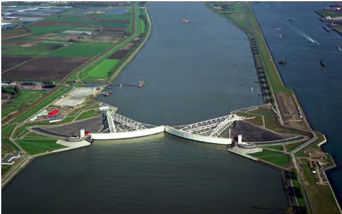
8. The surge barrier of Maeslantkering on the confluence of the rivers Oude Maas and Nieuwe Maas, Netherlands (opened on May 10 th , 1997, after six years of construction)
