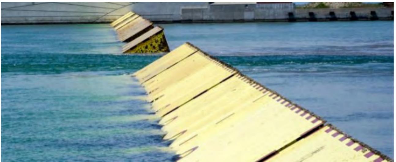
6. Mobile dams (note the defective and not working dam)
